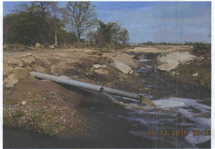
Right bank looking Northwest at two 6" outlet pipes
