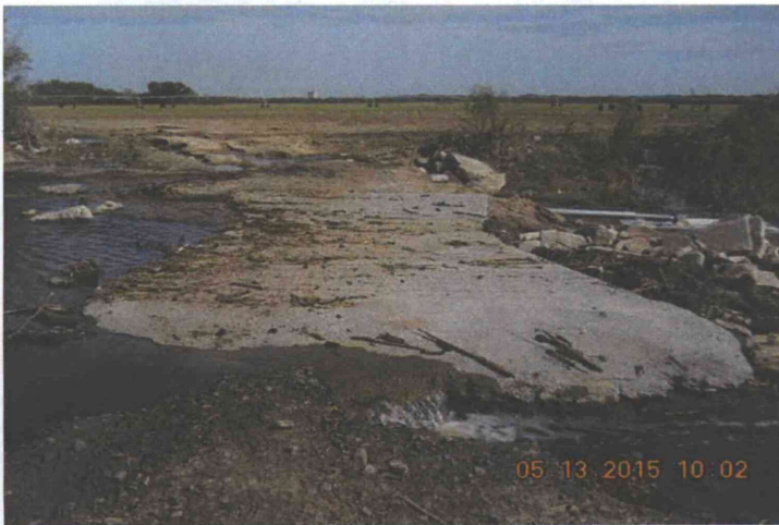
Right bank looking North
