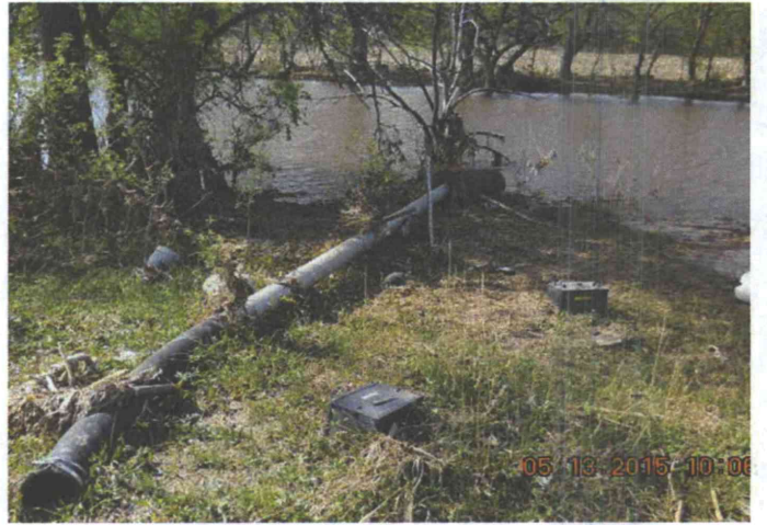
Diversion equipment on left bank at pumpsite
